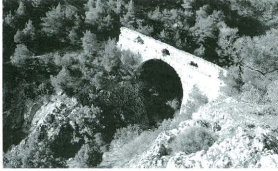
Fig. 12 Kemerköy aqueduct in the Kemerdere valley which was constructed to channel water collected from the southern slope (right) to the north (See fig. 4).
